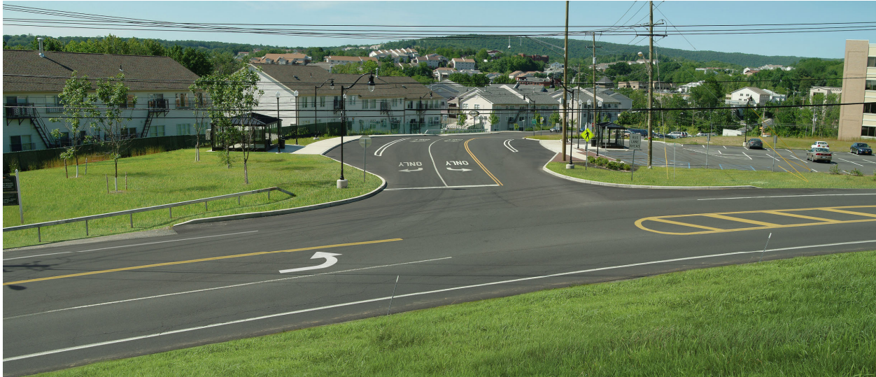
Roadway and Sidewalk Improvements
